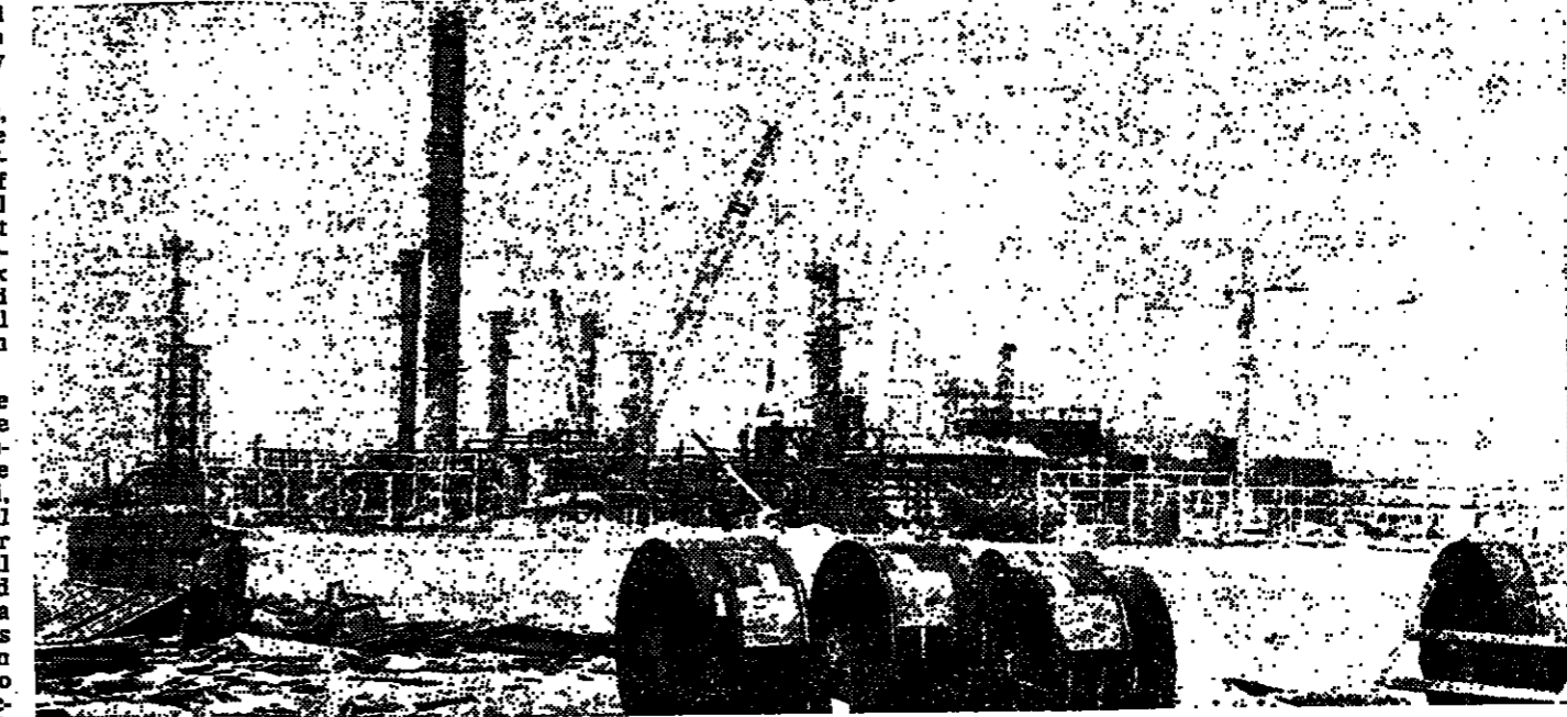
Qatar's first petrochemical plant under construction at Umm Said. It is scheduled for completion by 1980
